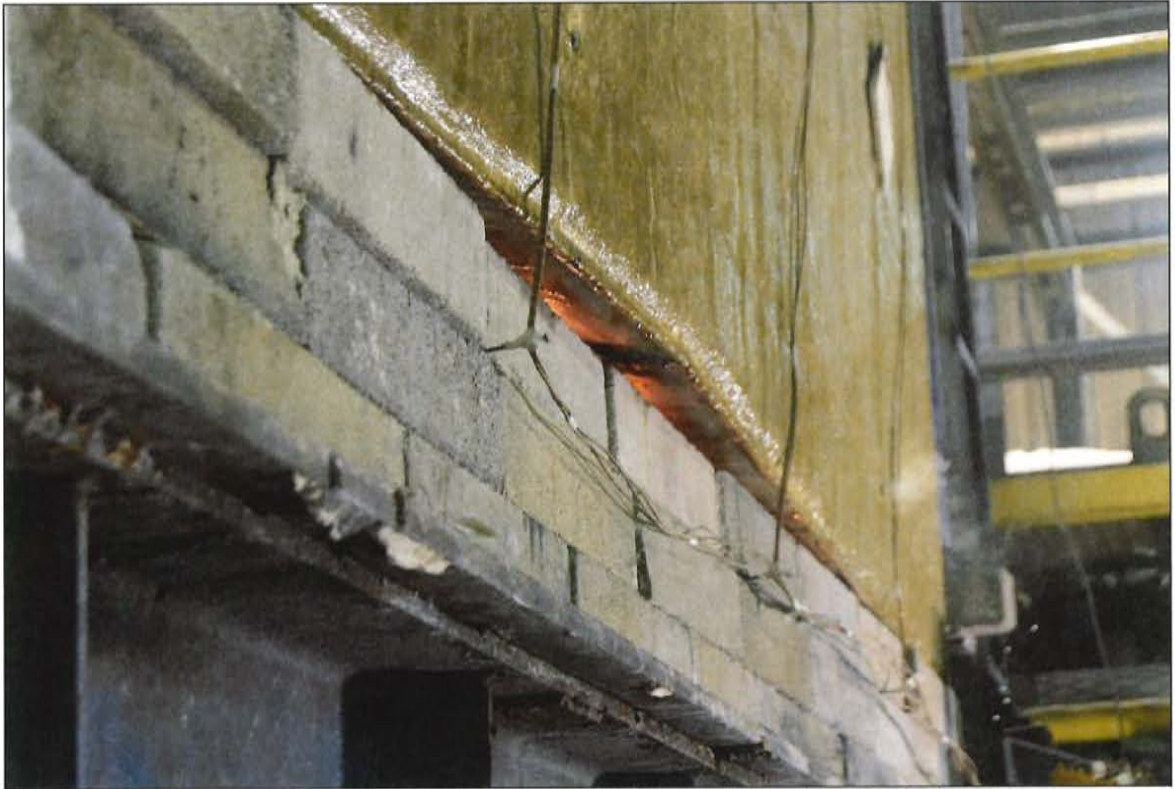
Figure C-5. Lower Edge of Serial No. 4001b Wall Assembly 29 min into Test.
