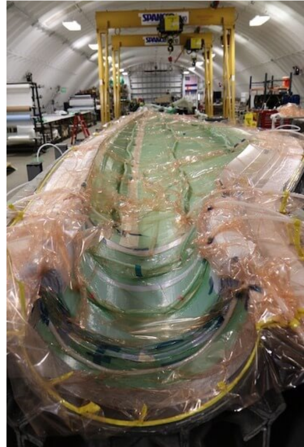
Construction of a revolutionary 13-meter thermoplastic blade at NREL. A vacuum bag covers the laminate and mold, which is infused with resin.
