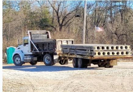
Ship to site
